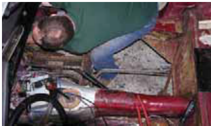
8. After removing as much as possible with the body saw, we attacked the spot welds with an air chisel. We put the chisel between the remaining floor pan sheetmetal and the body sheetmetal. (Be careful not to cut the latter.)
