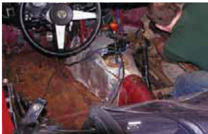
9. Once all of the pan was out, we ground all of the spot welds smooth and sanded the rusty metal.
